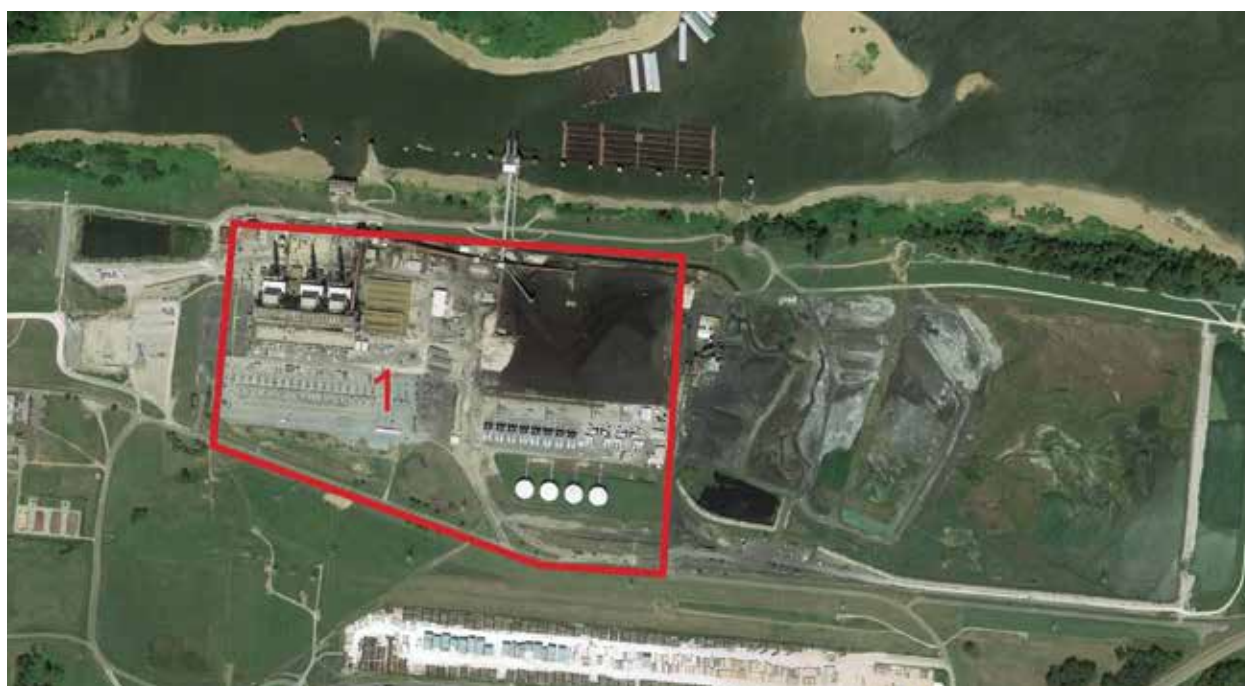
TVA Steam Plant
